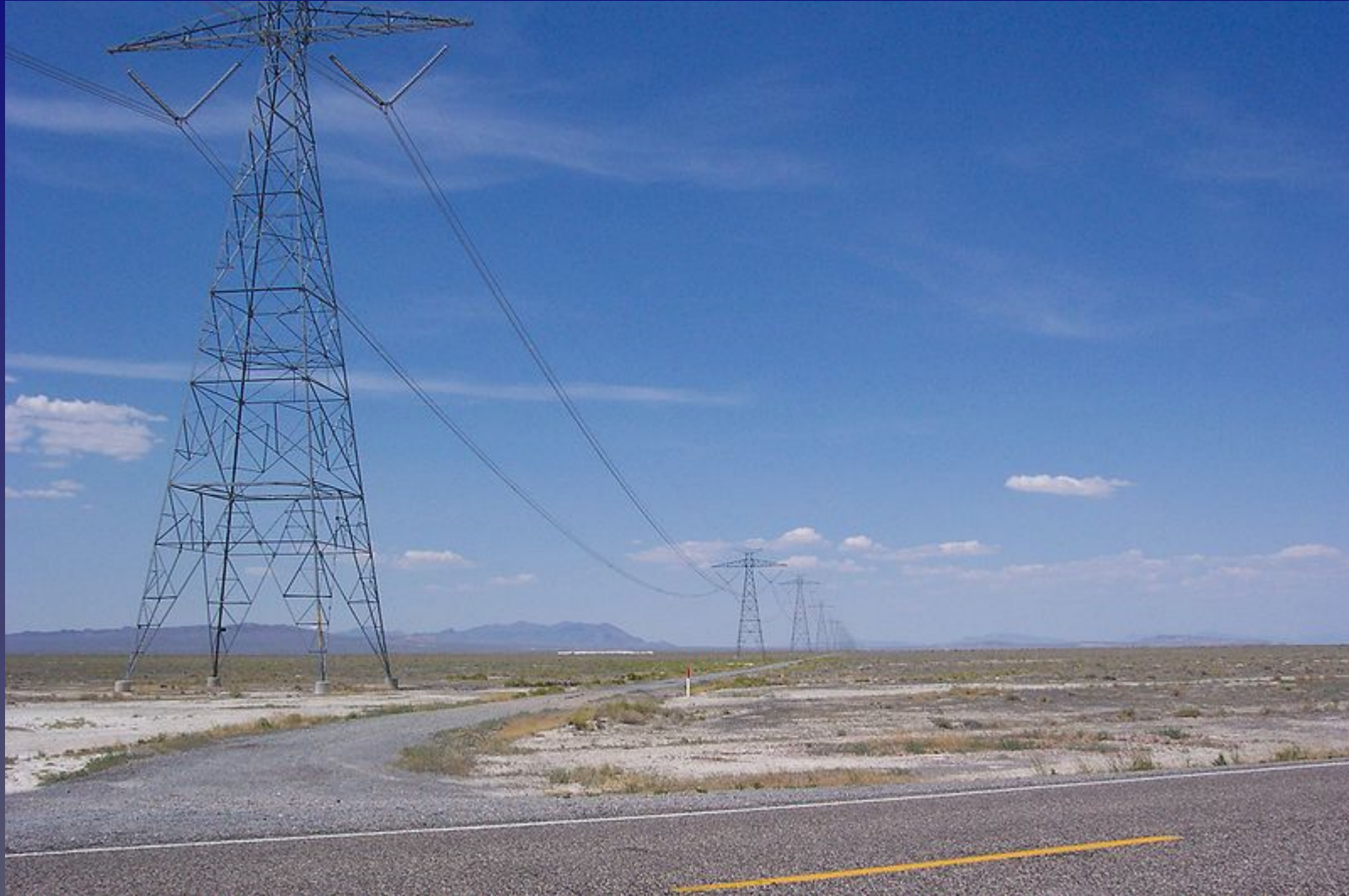
The Intermountain DC transmission line in Utah, \pm 500\text{kV}
